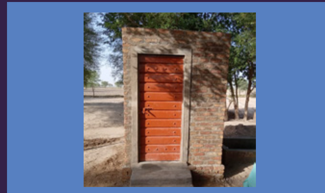
21,428 sanitations facilities were installed
